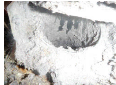
Disconnected Branch Duct; Missing Register
