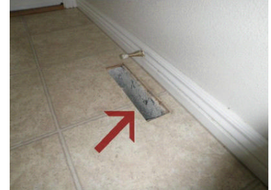
Disconnected Branch Duct; Missing Register
